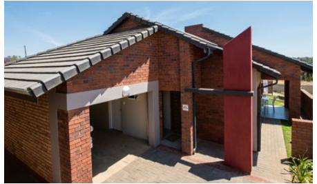
A flat profiled tile delivers a sleek, modern roof.
